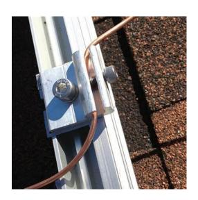
Slide a K-Nut into the rail's deep channel, positioning it under the chosen lug location. Set the grounding lug over the rail with the green barbed bolt facing the rail surface to ensure proper bonding. Insert the bolt with its washer through the lug and thread it into the K-Nut. Connect your copper grounding conductor to the lug's terminal, ensuring proper strain relief and routing along the rail.
